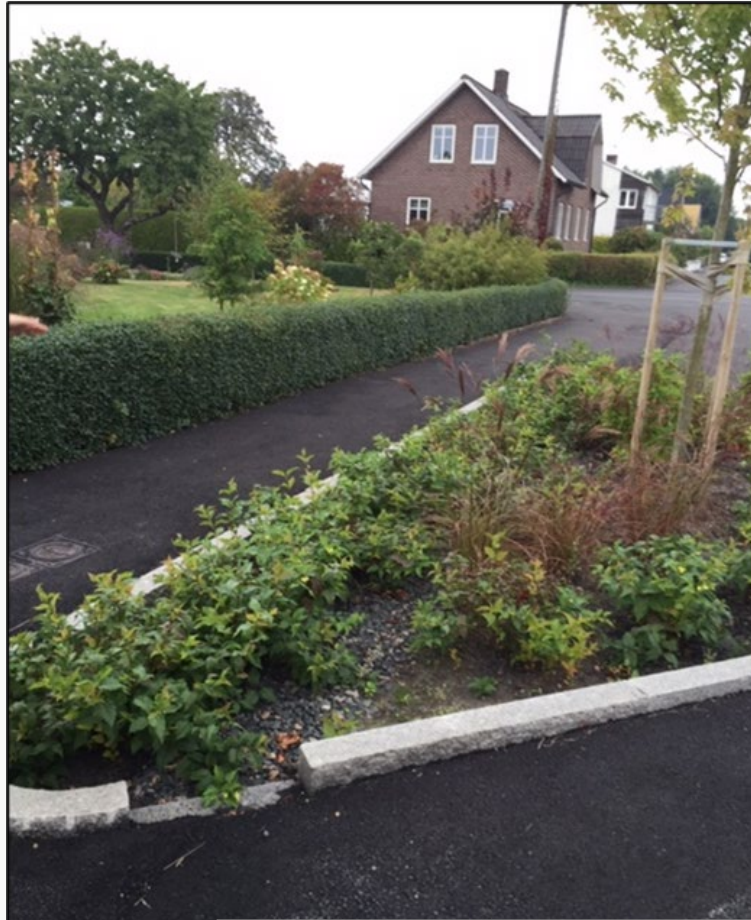
Biofilter, rainingarden mm
